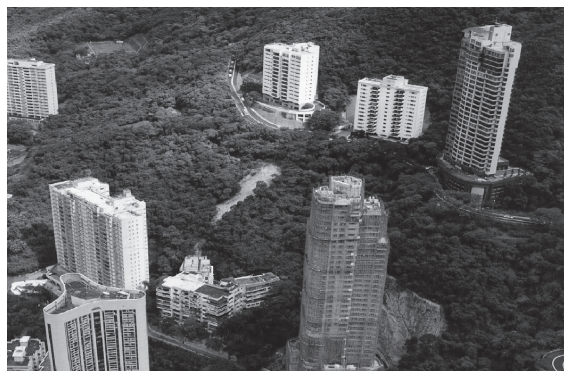
Figure 17. A 20 m 3 landslide in 1998 resulted in damage to property
