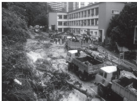
Figure 8. Liquefied debris of the 1992 Kennedy Road landslide
